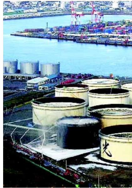
Photo-1. Fire of Oil Tank after the Earthquake
